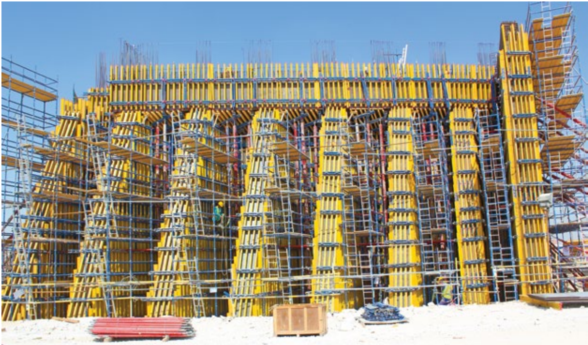
C. ABUTMENT FORMWORK WITH DYNAMIC H-20 PANELS
