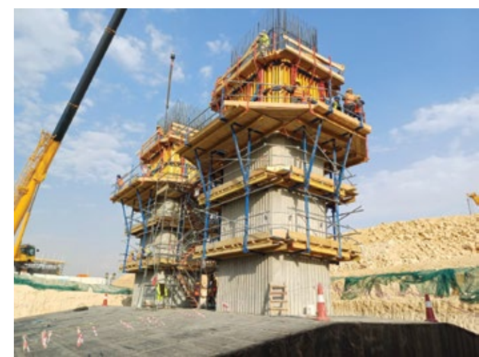
[B] BSC SELF-CLIMBING PLATFORM WITH DYNAMIC H-20 PANELS
