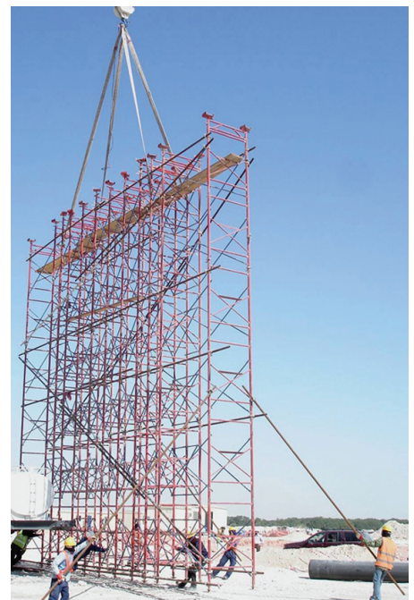
VERTICAL LIFTING BY CRANE
