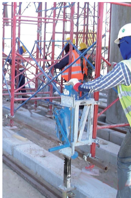
HORIZONTAL SHIFTING WITH TRANSPORTATION WHEEL JACK UNIT
