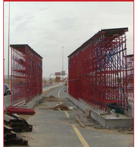
Shoring and Secondary beams
