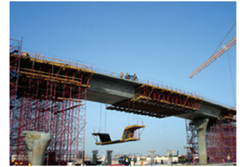
Acrow Bridge table form
