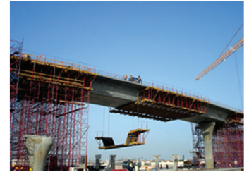
Acrow Bridge table form
