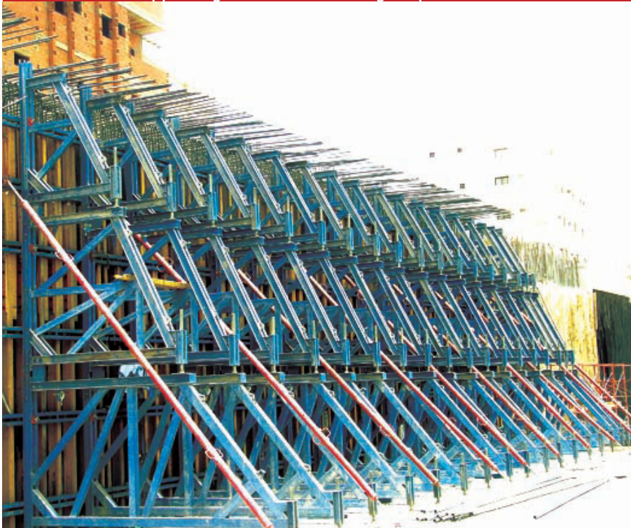
Supporting frame for wall height up to 7.60 m
