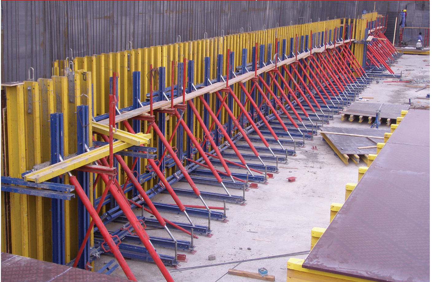
Supporting frame for wall height up to 7.60 m
